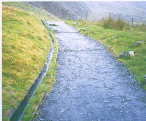
Locally imported stone not matching local geology - man made drainage material and path edging not hidden
