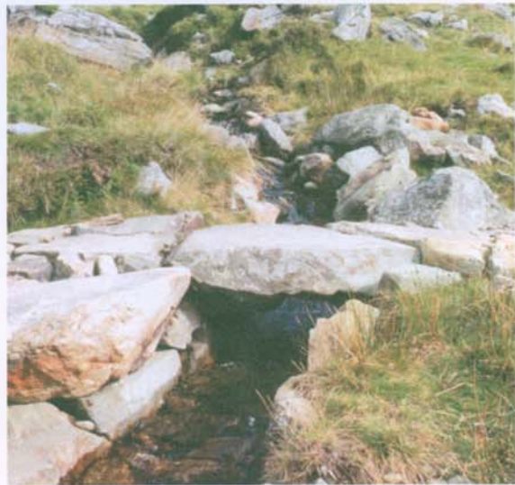
Locally derived stone successfully used for drainage
