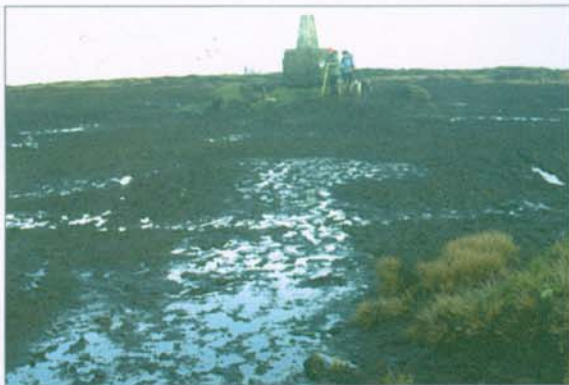
Obvious severe erosion
