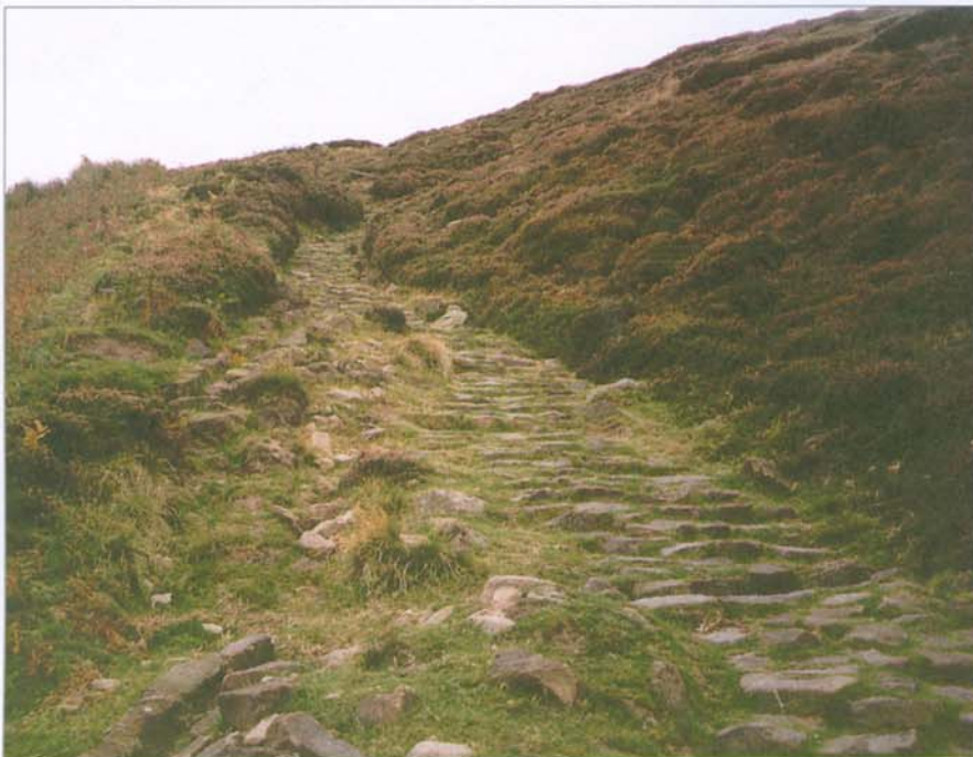
Investment protected by maintenance - with path use contained and erosion stabilised
