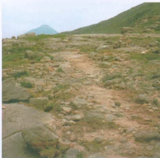
Major repairs pre-empted - loose stone removed to define an improved surface
