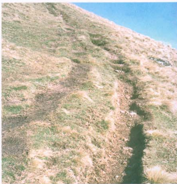
Problem developing - drainage control and vegetation support needed
