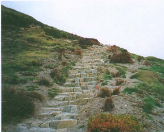
Stepping not avoided, unsuitable uniform stone used and path edges insensitively landscaped
