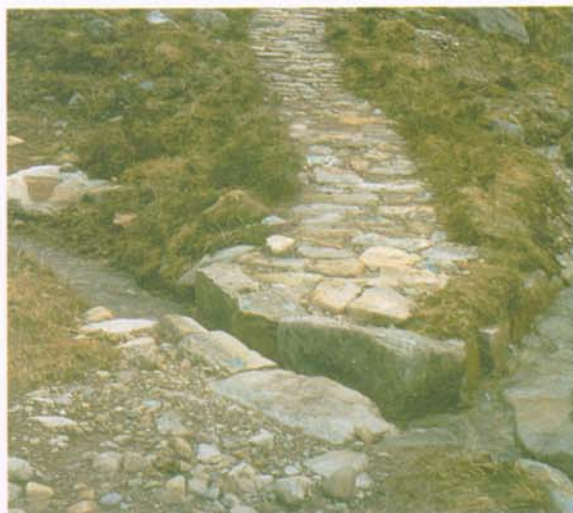
Good design and construction of adequate size drain
