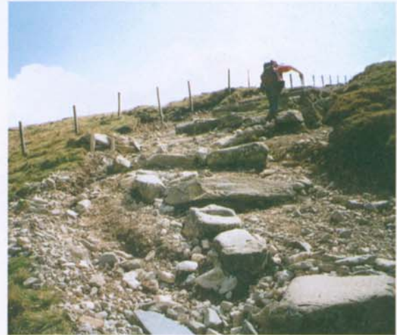
Lack of maintenance - erosion not stabilised and further major works needed
