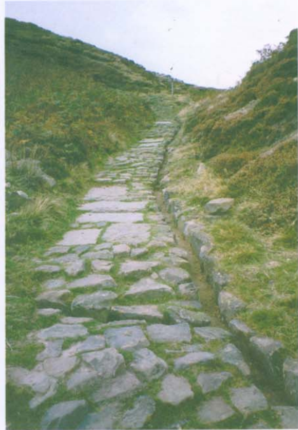
Evidence of after-care maintenance
