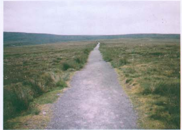
Unsuitable uniformity of path surface, width and line
