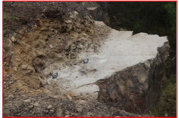
Bolts recently placed at Egerton Quarry
