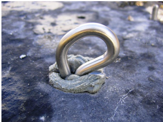
After testing to 20kN
