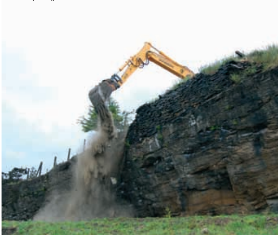
Recent BMC conservation work(!) at Craig y Longridge. Photo: Guy Keating.
